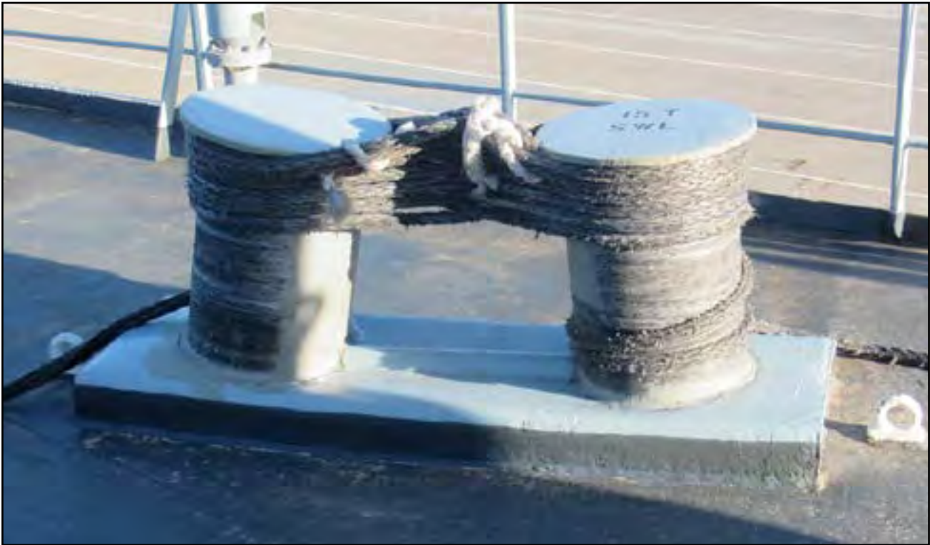
Figure 2: Damage to mooring bitts following surging alongside berth
