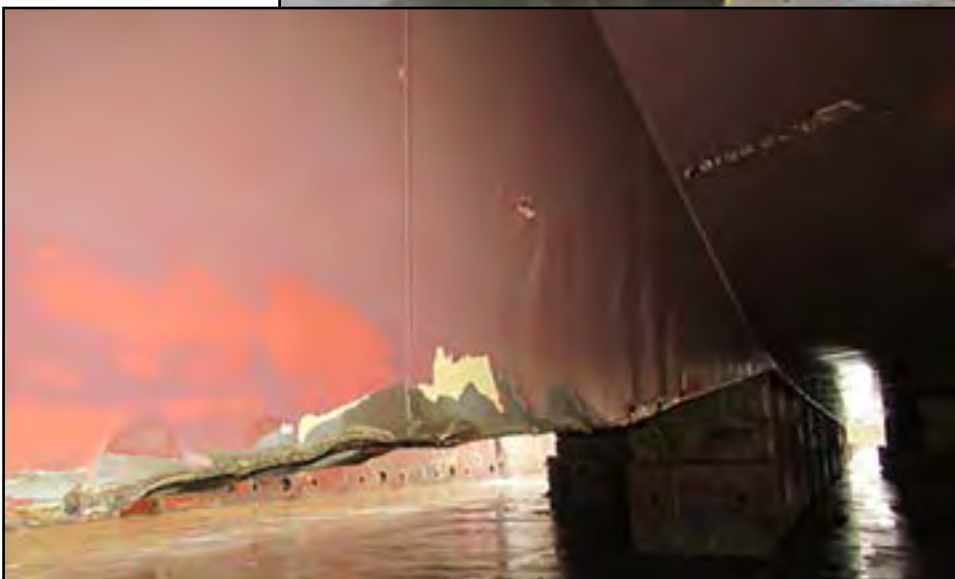
Figure: Damage to skag
